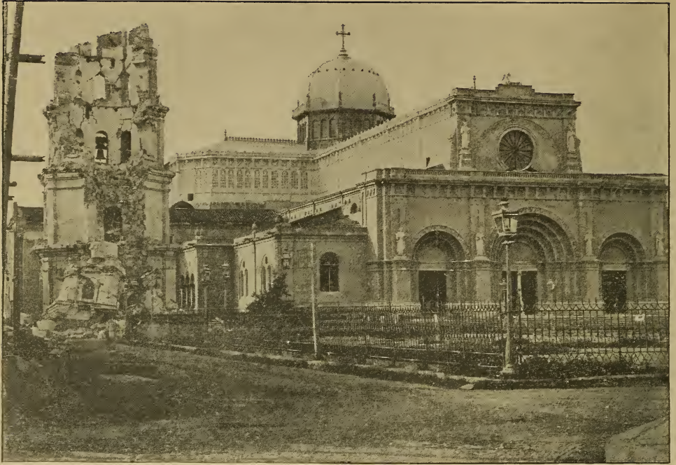
CATHEDRAL OF MANILA AFTER EARTHQUAKE.
